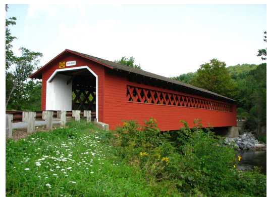
Henry Bridge, Bennington Bill Caswell Photo
